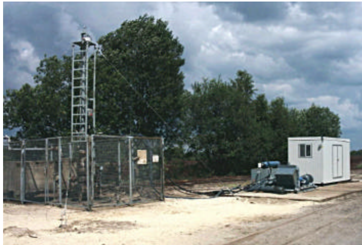
Figure 3: The mast of the pulsing tool with the hydraulic unit in the background.
